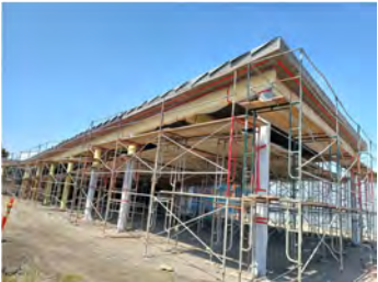
Outdoor Dining Area Installing the stucco on the canopy
